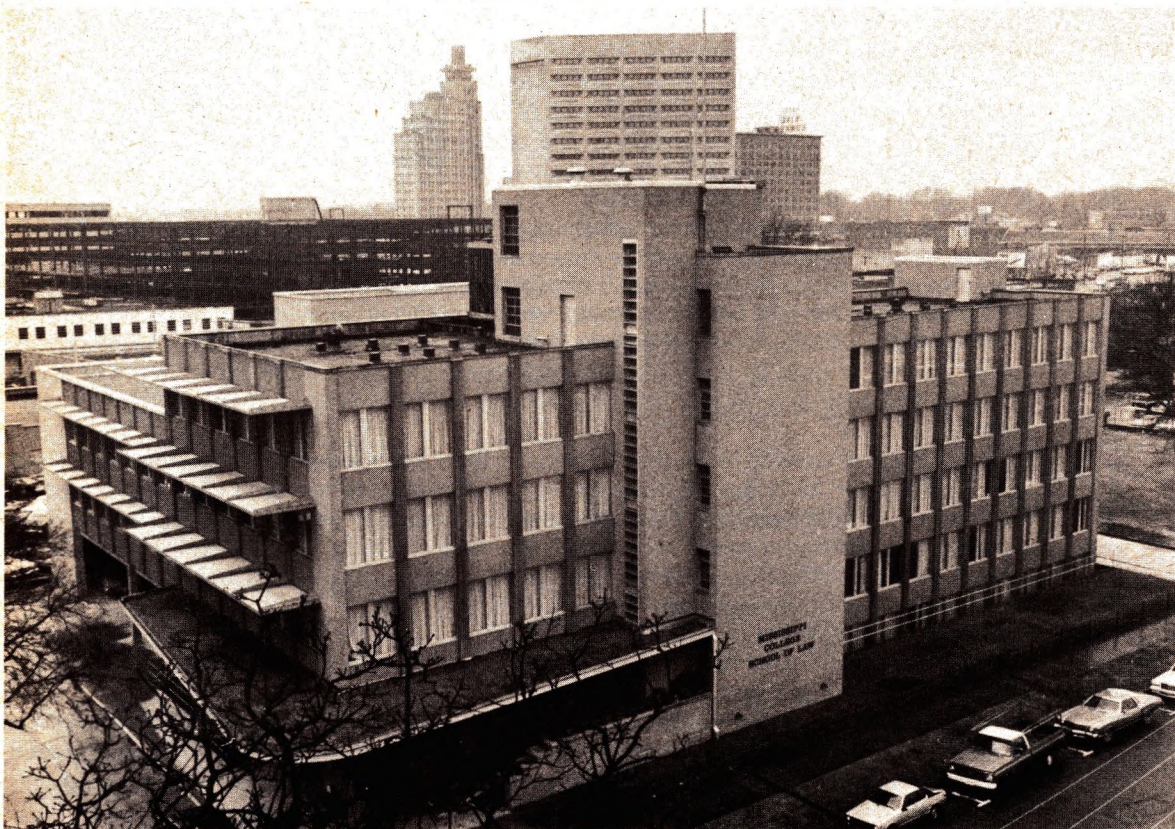
MISSISSIPPI COLLEGE SCHOOL OF LAW located in Jackson, Mississippi, site of PAD's 163rd chapter which was installed August 6, 1980. The story appeared in December, 1980 issue of The Reporter .
