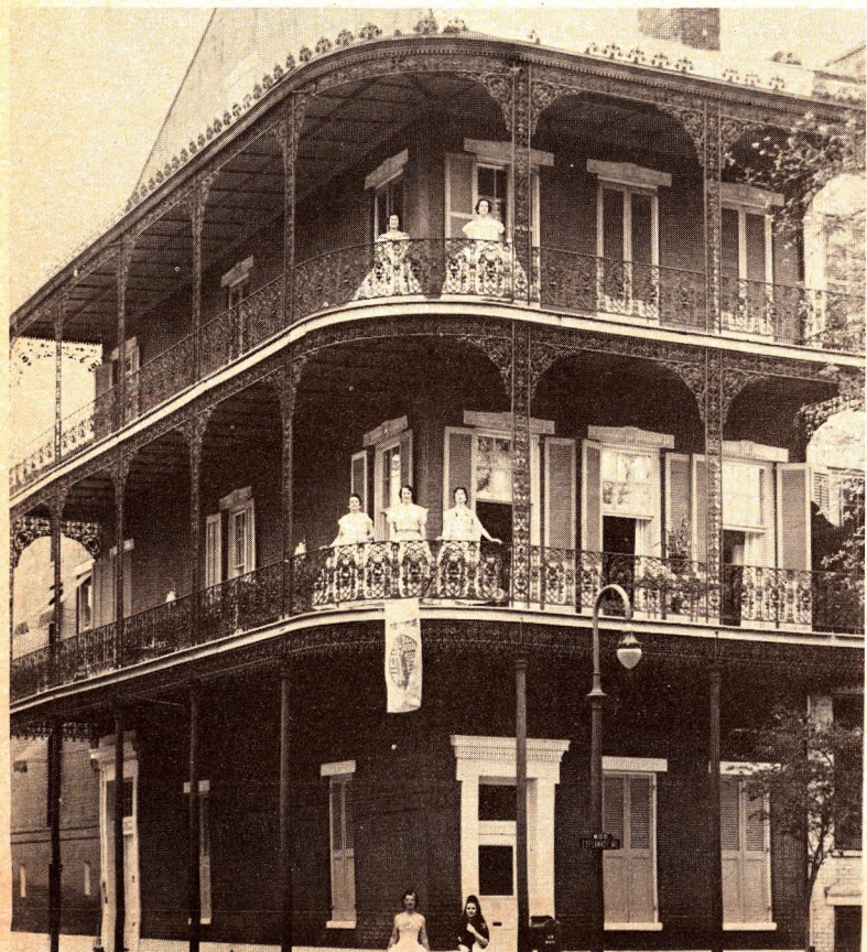
TYPICAL NEW ORLEANS FRENCH QUARTER HOME — Set with balcony decorated in wrought and cast iron, this typical New Orleans French Quarter home recalls the appearance of New Orleans when the city was a colony of Spain during the 18th century.
